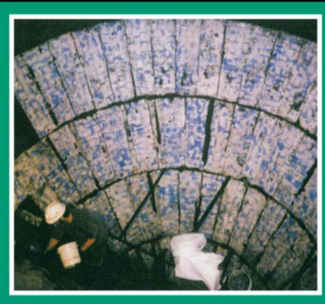
Pre-engineered WearSpan® panels being installed in a badly worn coal load-out hopper 22' in diameter.
