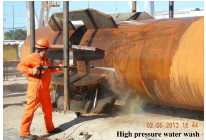
Surface preparation – simple and inexpensive
